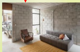
EXPOSED BLOCK WALL
