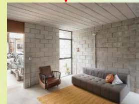
EXPOSED BLOCK WALL
